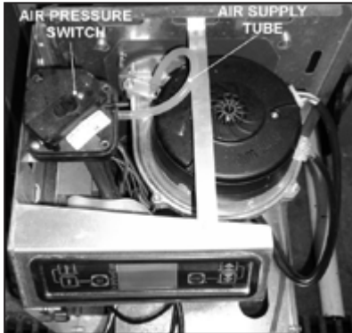
Figure 12-7: Air pressure switch and fan
