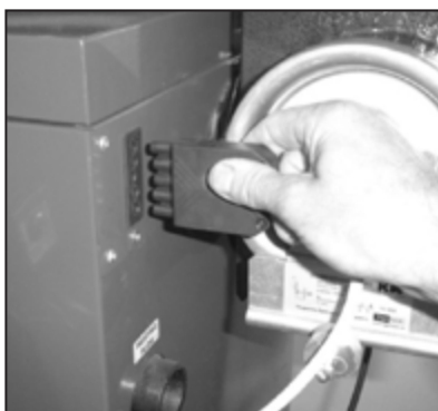
Figure 11-2: Disconnecting fan/solenoid 5-way plug
