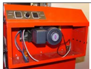
Figure 10-2: Boiler control panel (cover removed)
