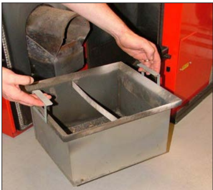
Figure 10-7: Lifting ash pan using carrying handles
