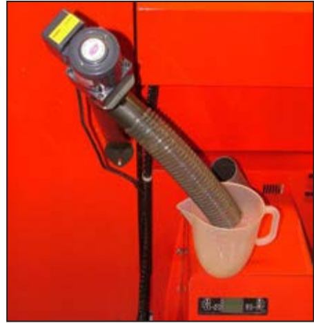
Figure 7-3: Pellet tube ready for priming the pellet auger
