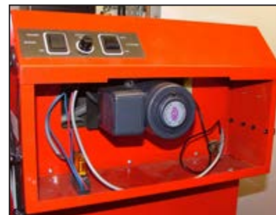
Figure 11-6: Boiler control panel (cover removed)
