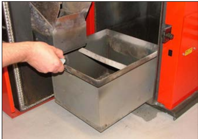
Figure 10-6: Removal of ash pan from boiler
