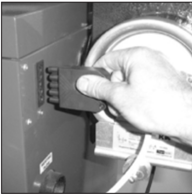
Figure 8-2: Flue fan/solenoid valve plug connection
