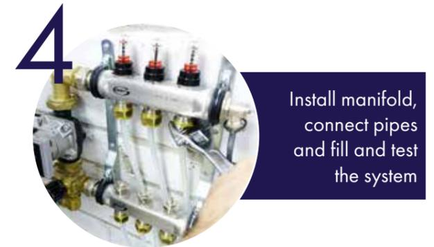
Install manifold, connect pipes and fill and test the system
