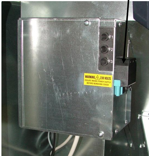
Figure 8-1. Wiring centre
