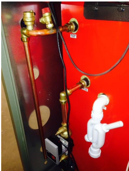
Figure 6-1. Sealed system kit
